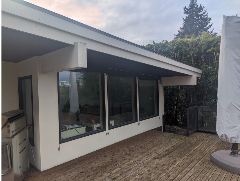
EXISTING WALL WHERE PERGOLA IS TO BE ATTACHED
